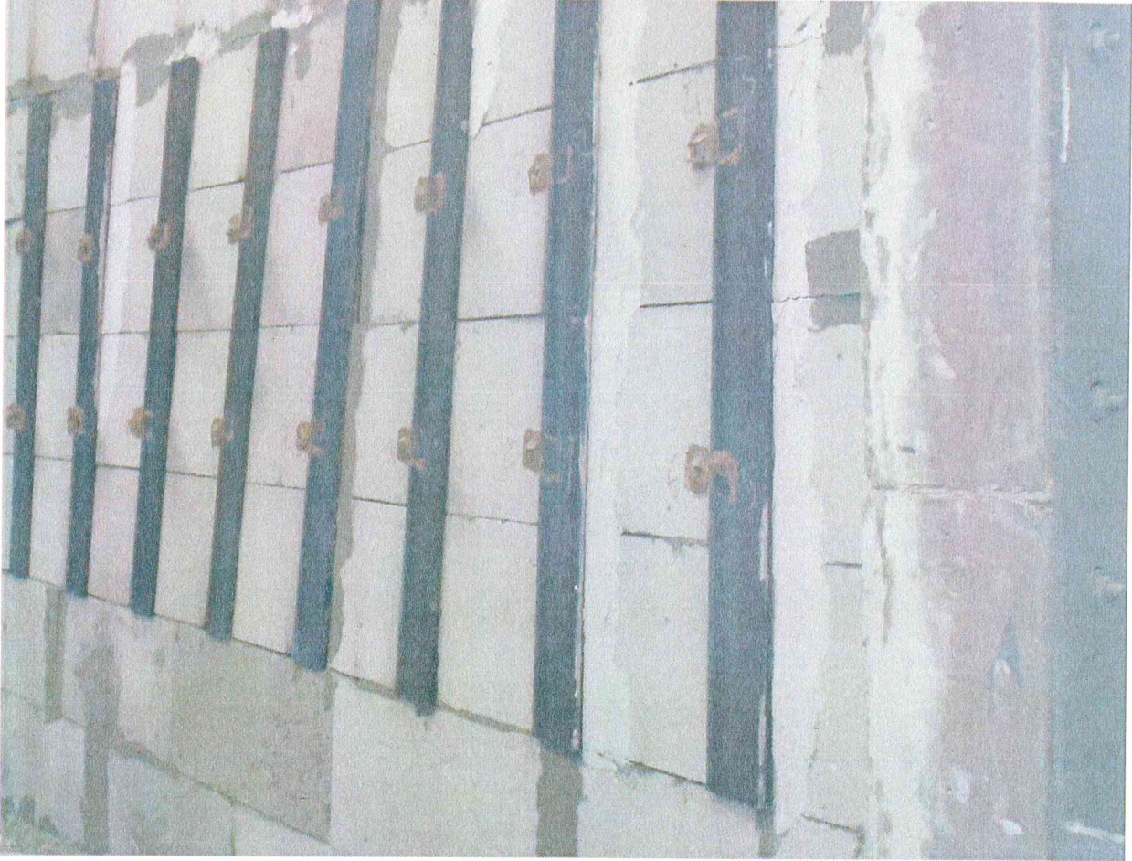
Photo C3: Unexposed side of the test specimens after the test.
